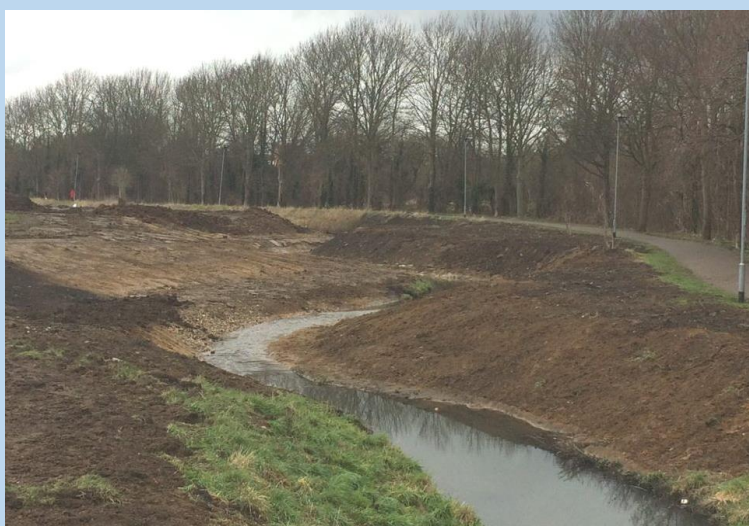
Figure 6-1 – New meanders adjacent to Larkspur Walk
